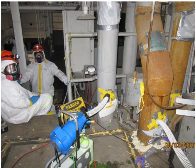
Ventilation Duct Application: Internal Stabilization
