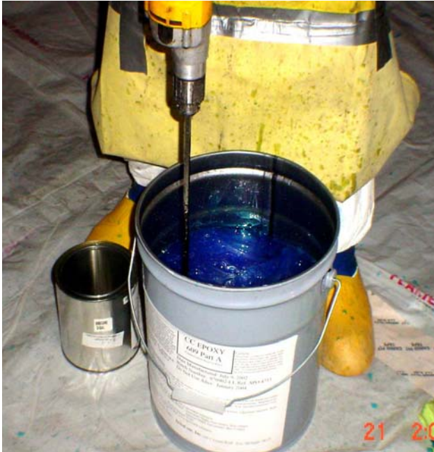
Mixing the resin and hardener
