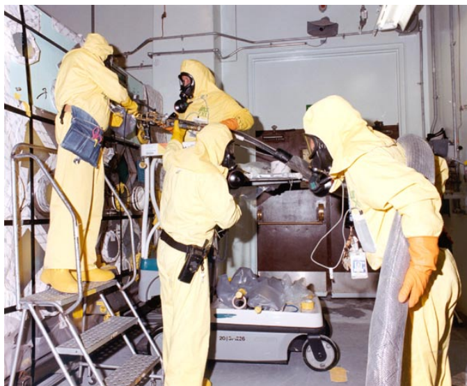
Workers spray structural expanding foam inside a glovebox at Rocky Flats. When hardened, the foam meets Envirocare acceptance criteria for crush resistance and integrity.
